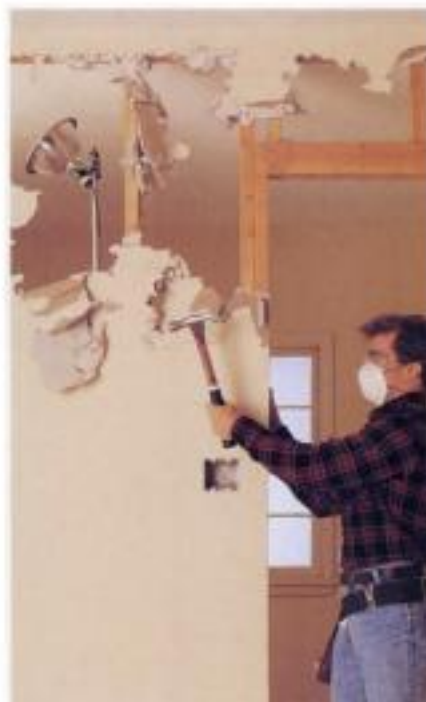
Removing interior partition walls between rooms is covered on pages 186 to 188.
