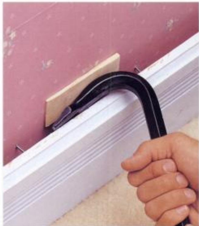
A wrecking bar , sometimes called a crowbar, is a rigid tool for demolition and heavy prying jobs. Use scrap wood under the bar to protect surfaces.
