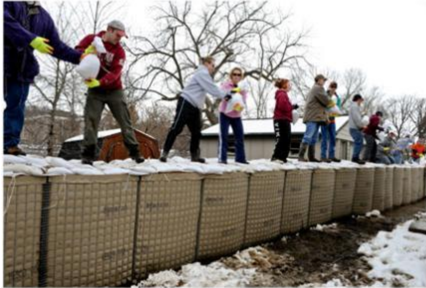
Figure 7 - Volunteers raising emergency levee in Valley City, North Dakota (Source: U.S. Army Corps of Engineers Digital Visual Library, 2011)
